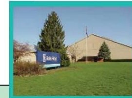
Rolls-Royce Energy Systems Inc. Mt. Vernon, Ohio 950 employees 400,044 sq. ft. Global HQ for the energy business, and design, manufacturing and packaging facility for industrial gas turbine compression and power systems
