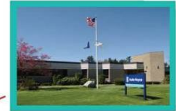
Rolls-Royce Naval Marine Inc. Walpole, Massachusetts 140 employees 121,000 sq. ft. Engineers and builds ship propulsion systems
